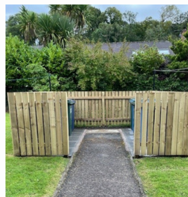
Bin area after
